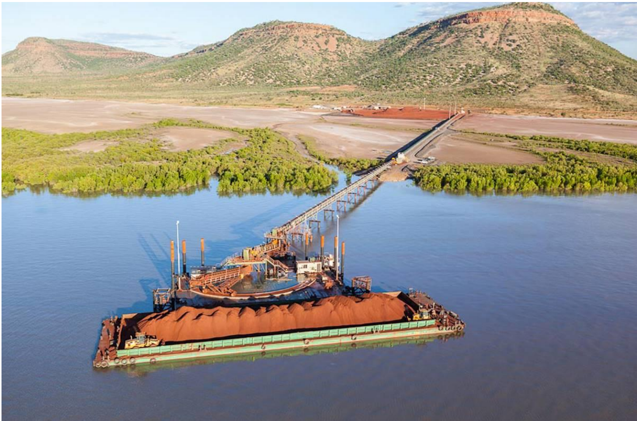
Figure 14 | Aerial view of an 'A' Frame jetty with ore loading onto a waiting barge or TSV
